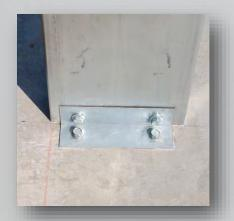
Structural steel buildings bolt to the foundation (slab, piers, strip) typically using cast in anchor bolts which are not supplied with the building kit.
