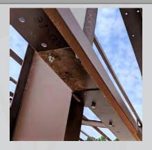
On site a Structural Steel main frame is typically bolted together with plates already welded in place in the factory. Structural Steel buildings can require some welding and drilling on site.
