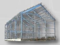
**Structural Steel** can be built at any size but start to be become more economical for spans over 50'. Ideal for very large spans (Walmart), tall buildings, buildings that need cranes, large unsupported overhangs, open riding arenas, large doors such as airplane hangers
