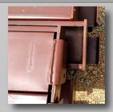
Structural steel has a painted finish typically in the red although can come in many colors. The paint is intended only to protect the steel during construction and transport and is easily damaged.
